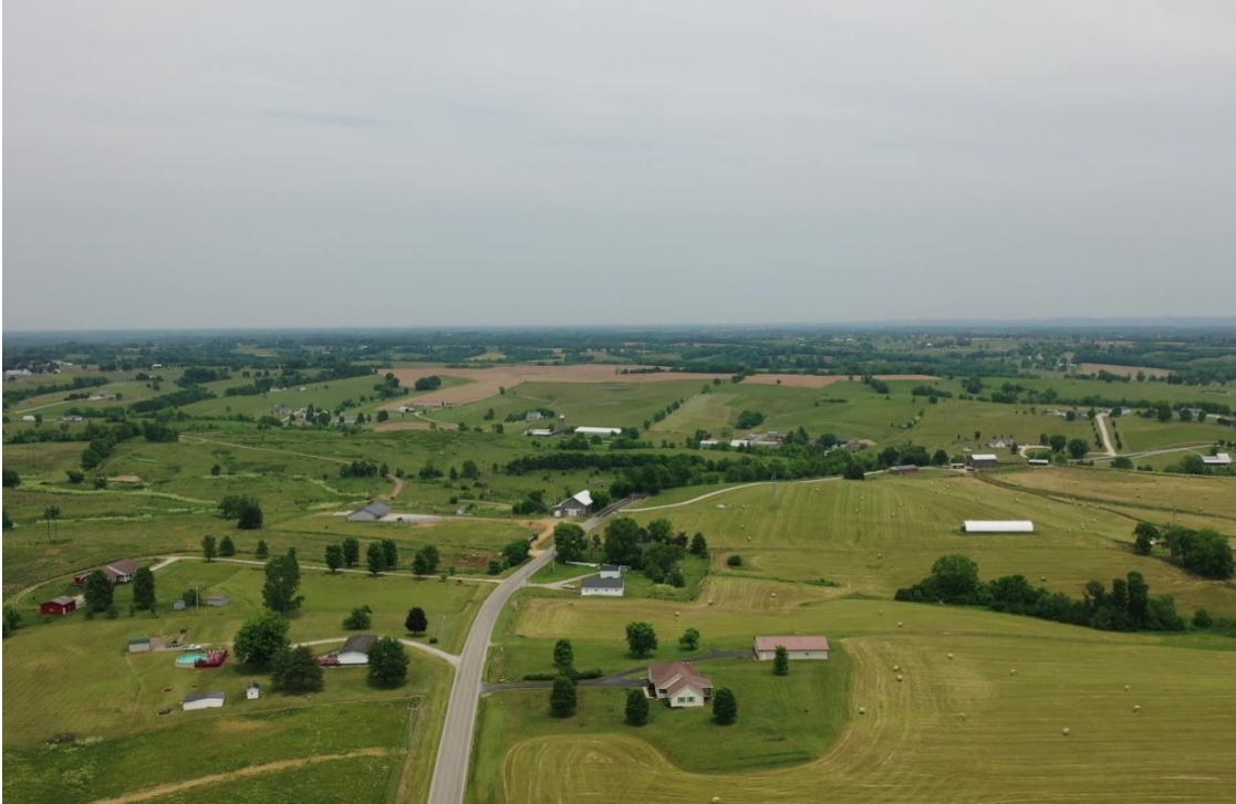
Aerial view of KY-57 between KY-3299 and KY-3301; looking north of KY-3301.
